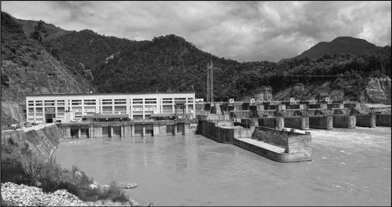
132 MW Teesta Low Dam-III Power Station (West Bengal) - Barrage
