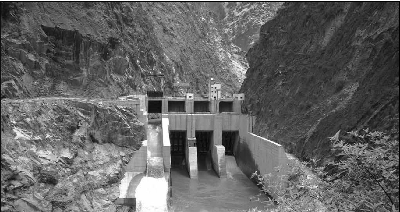
231 MW Chamera-III Power Station (Himachal Pradesh) - Dam
