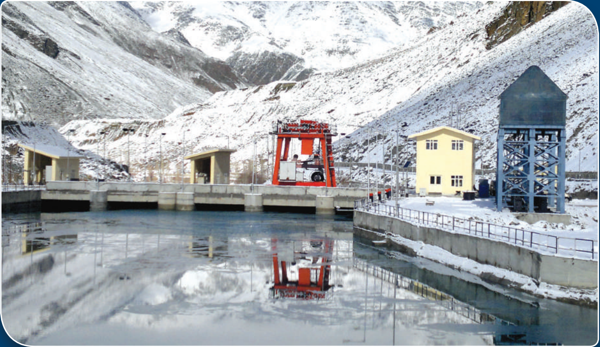
44 MW Chutak Power Station (J&K) - Dam
