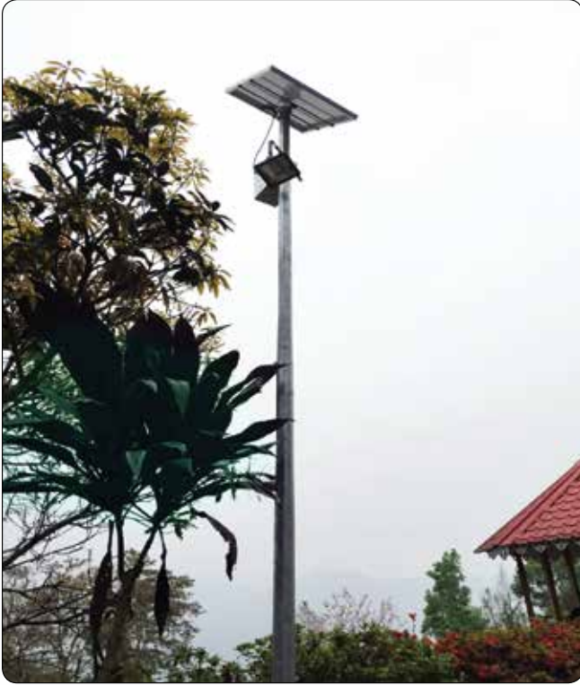
Installation of 15 nos Solar Street Lights at Mungpoo Outpost
