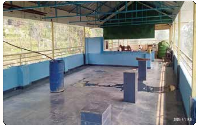
Construction of Steel truss fabrication at Makha Sr. Secondary School
