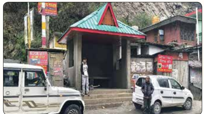
Construction of Rain Shelter in Gram Panchayat, Larji
