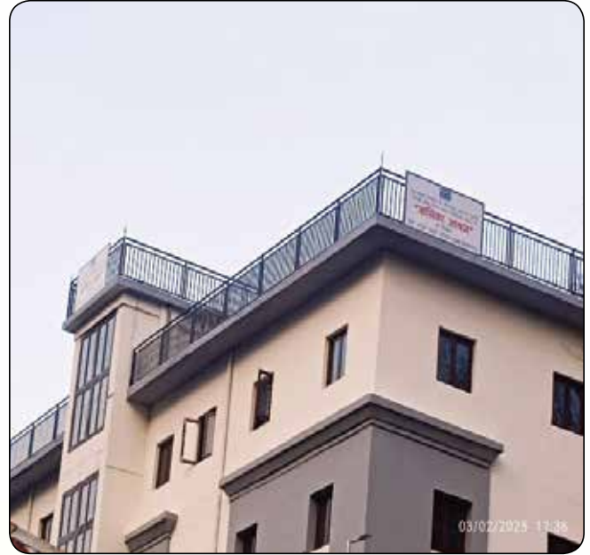
Construction of "BALIKA ASHRAM" Chilli, Tissa
