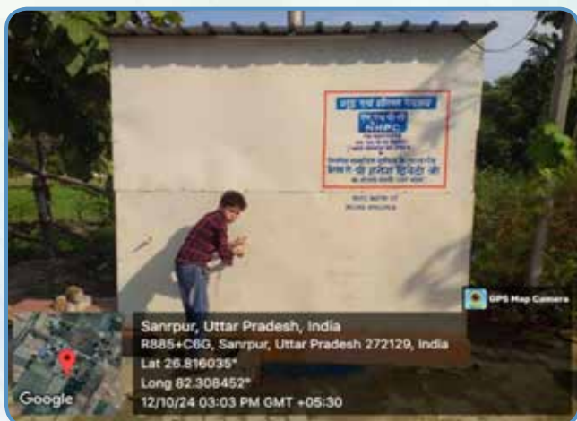
Installation of 10 Nos Reverse Osmosis (RO) Water System in District Basti of Uttar Pradesh
