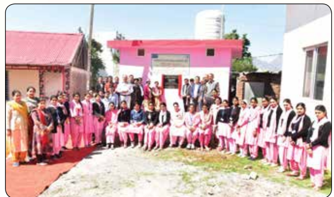
Construction of 02 Nos. Toilets at Industrial Training Institute, Reasi in Jammu & Kashmir
