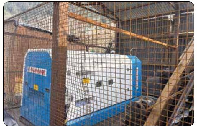
Installation of DG Set at PHC, Boniyar
