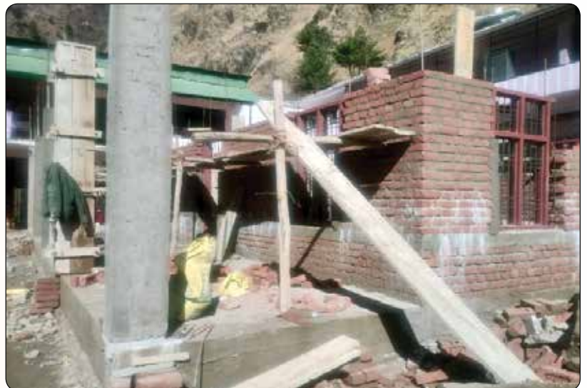
Construction of Two Rooms at Govt. Primary School Manikaran, Kullu
