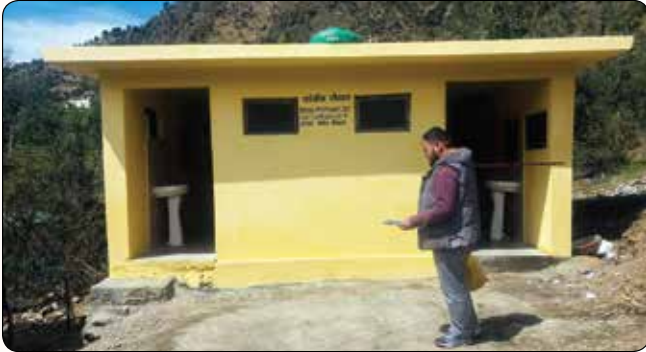
Construction of Toilet at GSSS Kohal
