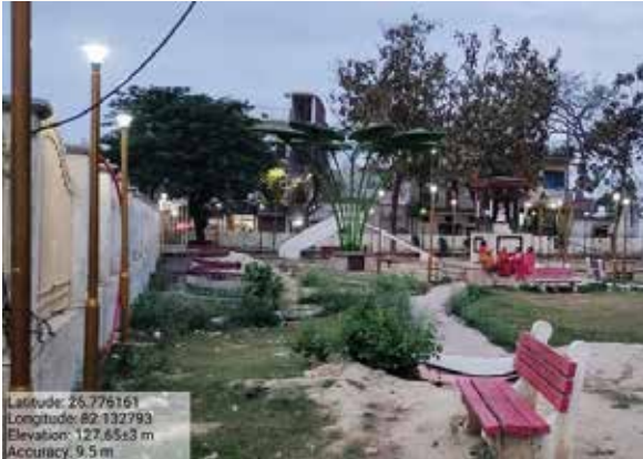
Development of 5 nos of Parks by providing Solar Trees and LED Lights in the holy city of Ayodhya, Uttar Pradesh through CSR
