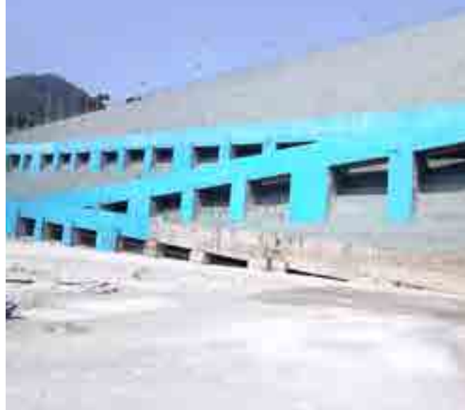
Fish Ladder at TLD-IV Power Station, West Bengal
