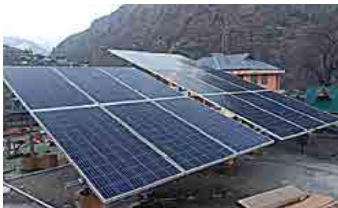
Installation of Grid Connected Roof Top Solar Plant
