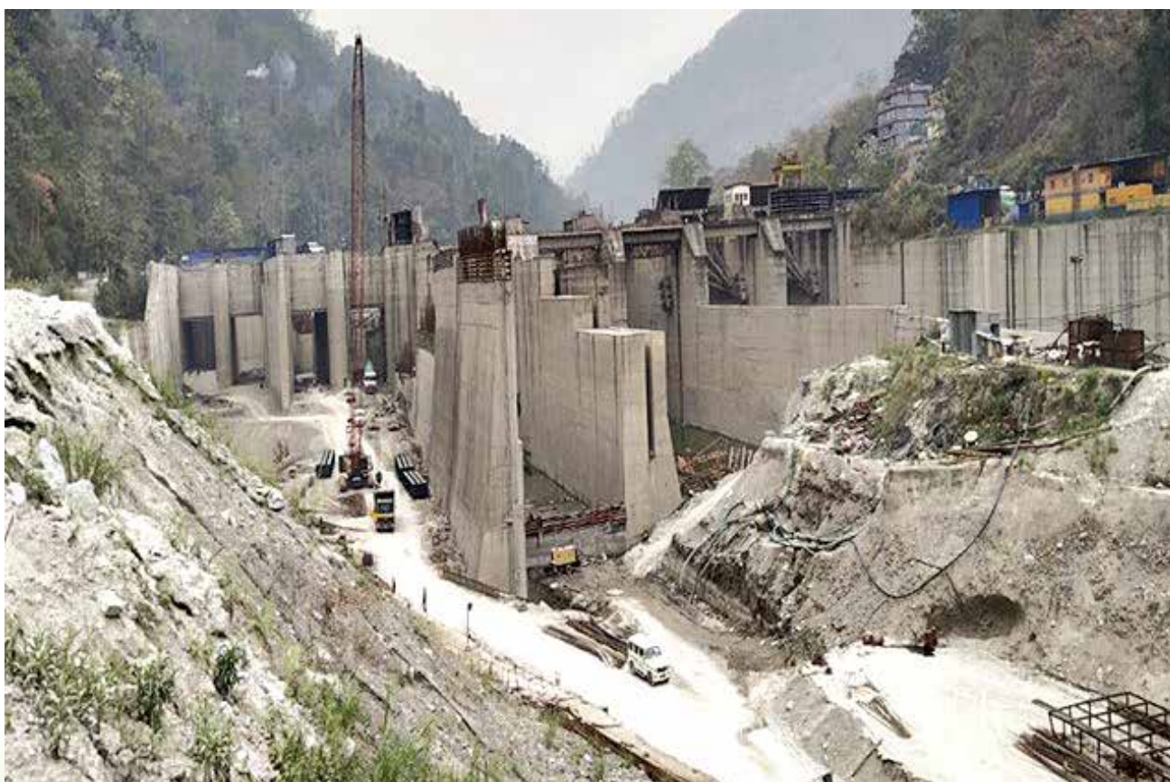
DOWNSTREAM VIEW OF BARRAGE – 500 MW TEESTA-VI PROJECT (SIKKIM)
