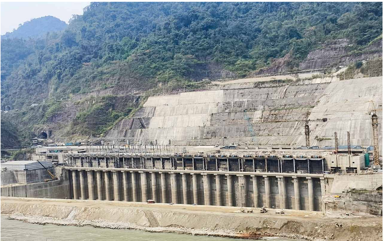
VIEW OF TAIL RACE CHANNEL AND DRAFT TUBE GATES - 2000 MW SUBANSIRI LOWER PROJECT (ARUNACHAL PRADESH)
