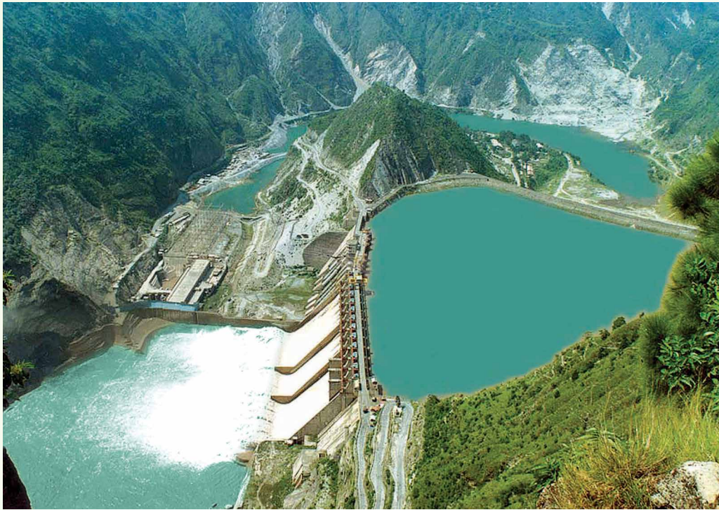
690 MW Salal Power Station (Jammu & Kashmir) - Dam
