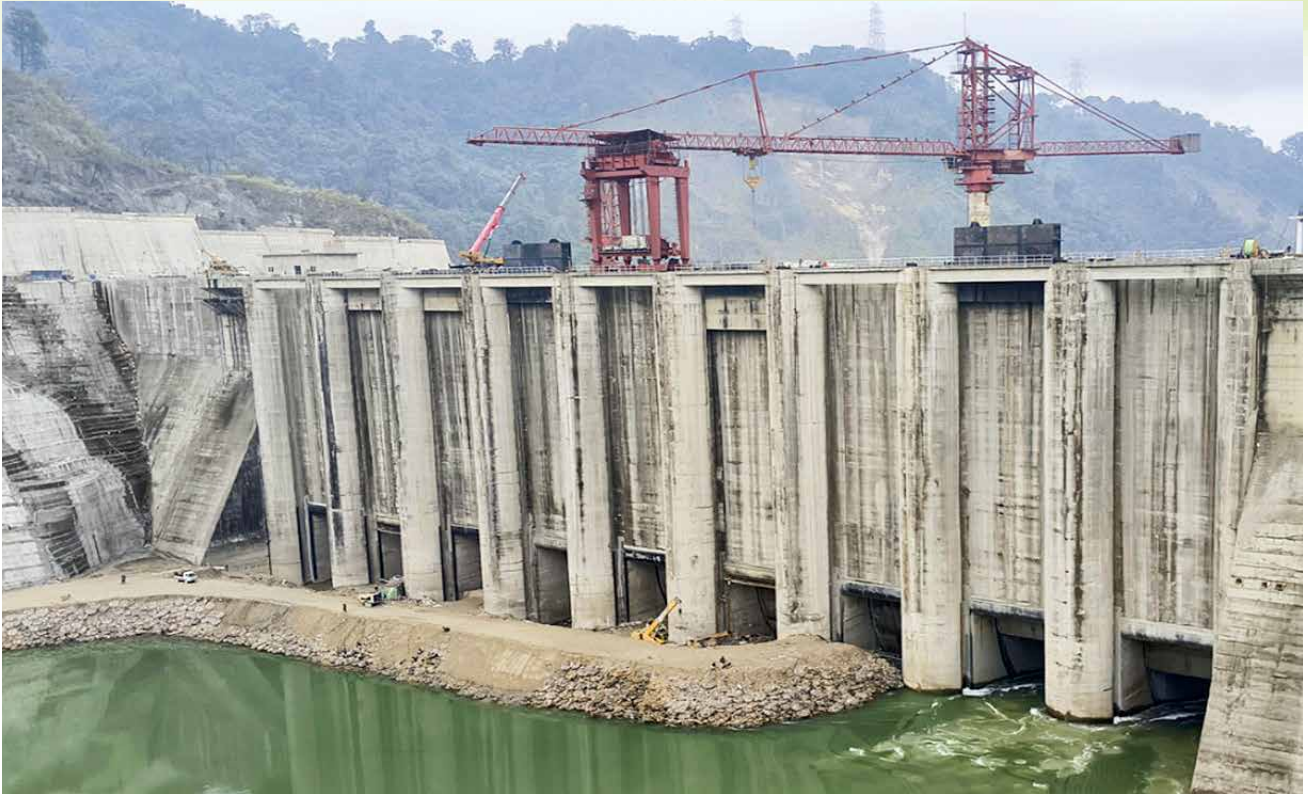
116 M HIGH CONCRETE GRAVITY DAM (UPSTREAM VIEW) – 2000 MW SUBANSIRI LOWER PROJECT (ARUNACHAL PRADESH)
