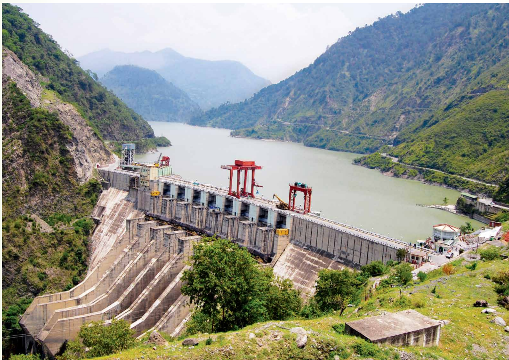
540 MW Chamera - I Power Station (Himachal Pradesh) - Dam
