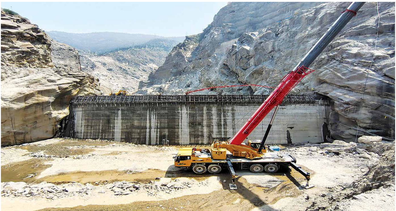
CONSTRUCTION OF COFFER DAM – 850 MW RATLE PROJECT (UT OF J&K)
