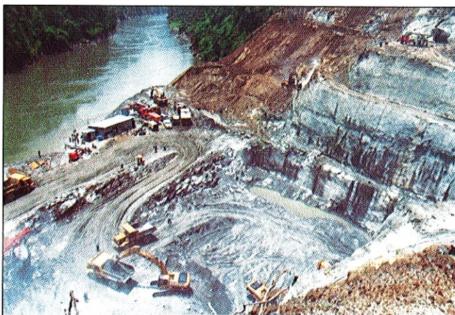
2000 MW Subansiri Lower Project (Arunachal Pradesh) - Diversion Tunnel Inlets at Dam site
