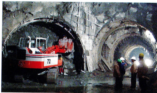
800 MW Parbati Stage - II Project (Himachal Pradesh) - Junction of bottom adit to Pressure shaft & Penstocks.
