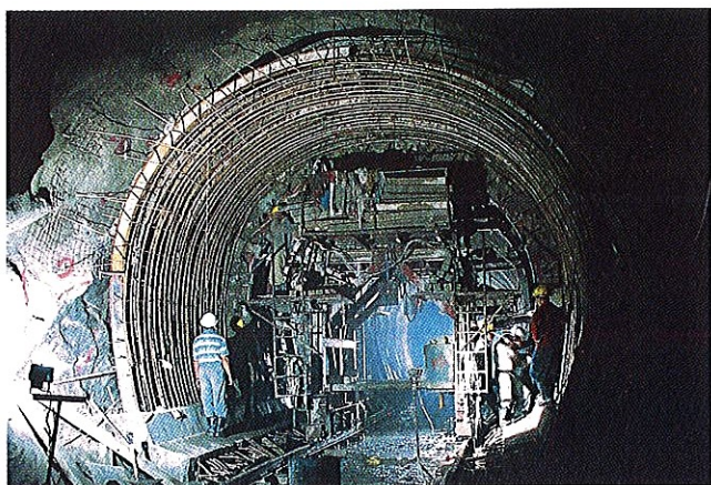
280 MW Dhauliganga Project (Uttarakhand) - Concrete lining of Intake Tunnel
