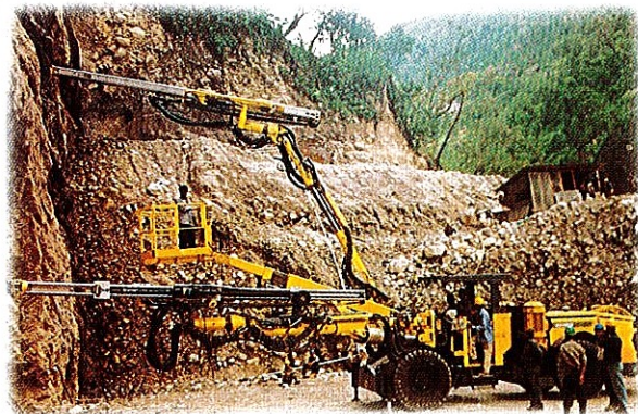
510 MW Teesta H.E. Project Stage-V - Sikkim (Drilling Operation at inlet to Diversion Tunnel)
