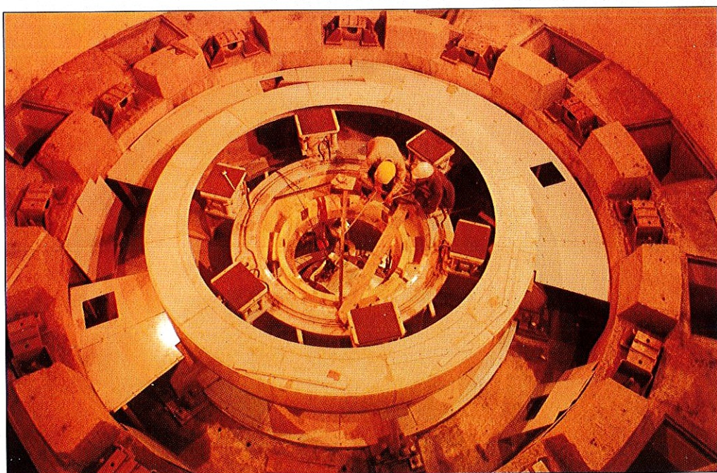
390 MW Dul Hasti Project (J&K) - Installation of lower bracket for unit-I in Power House
