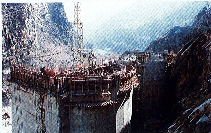
390 MW Dul Hasti Project (Jammu & Kashmir) Intake to Power Tunnel under construction
