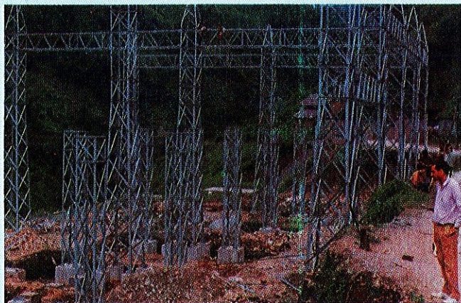
60 MW Rangit Project (Sikkim) - Erection of switchyard structure
