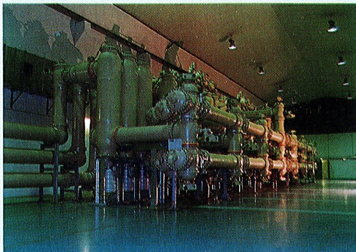
480 MW Uri Project (J & K) - Gas insulated switchgear
