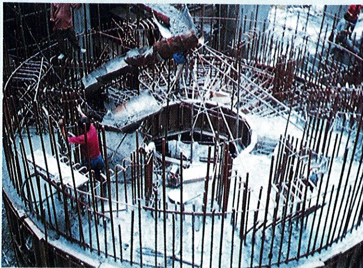
60 MW Rangit Project (Sikkim) - Erection of generator barrel of unit - 2
