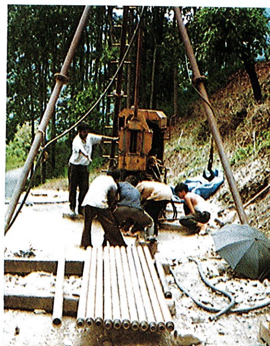
510 MW Teesta Project (Stage-V) - Exploratory drilling in progress at Surge Shaft location
