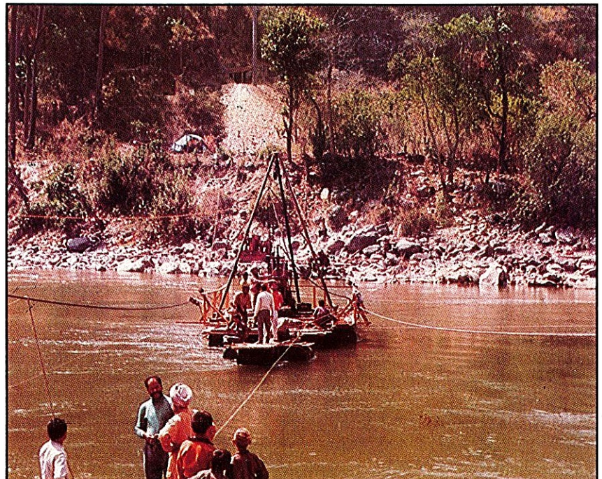
Investigation work in Progress - Kurichu Project
