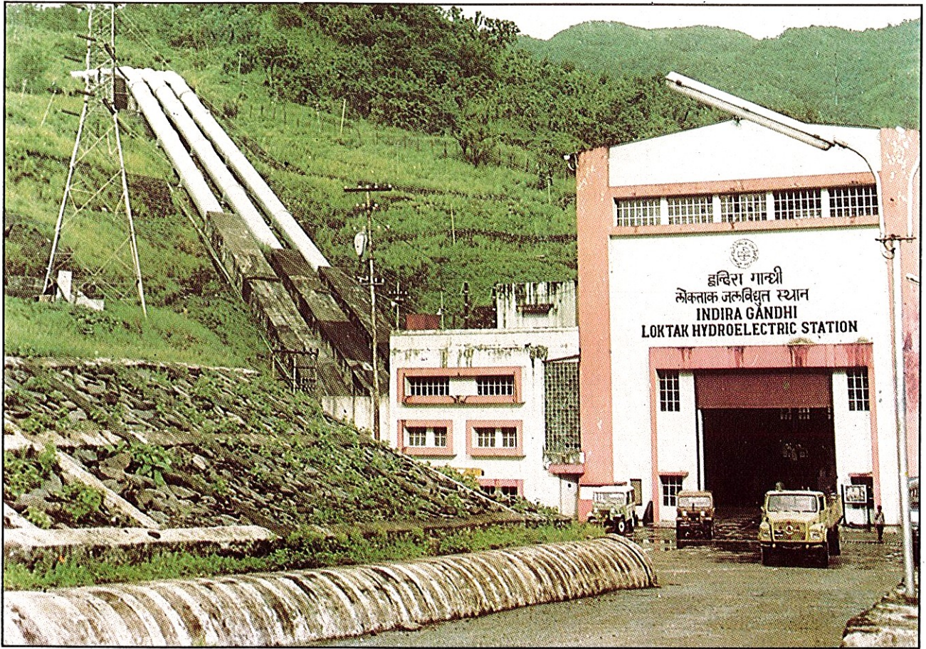
Power House - Loktak Project
