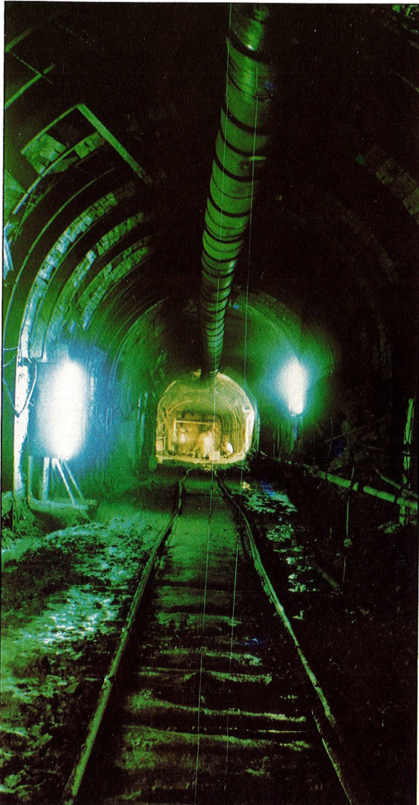
Tunnel under construction - Uri Project
