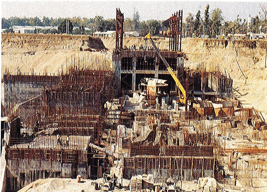
Tanakpur Project—Power House under construction
