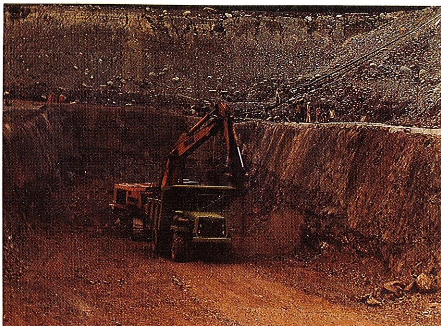
Excavation of Tail Race Tunnel—Chamera Project (H.P.).
