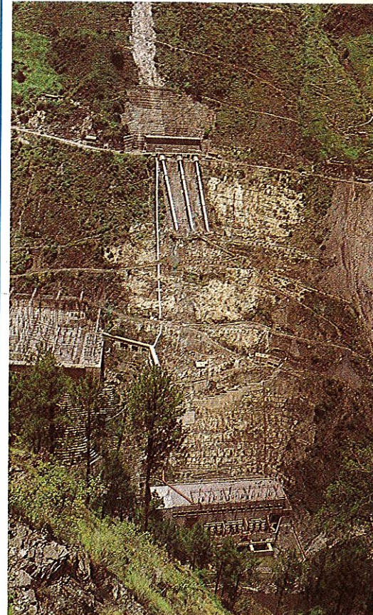
An Overview of power station complex-Baira Siul
