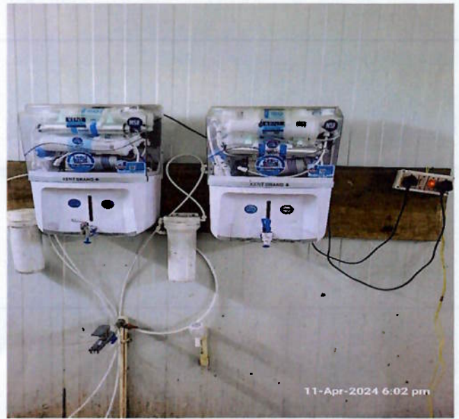
Fig iv: Image of RO Plant installed at site and camp.
