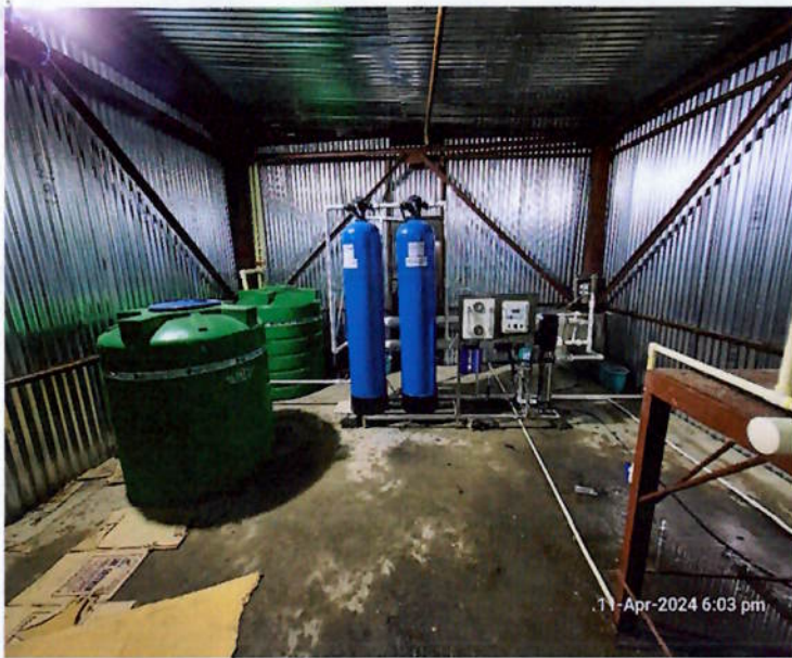
Fig iv: Image of RO Plant installed at site and camp.
