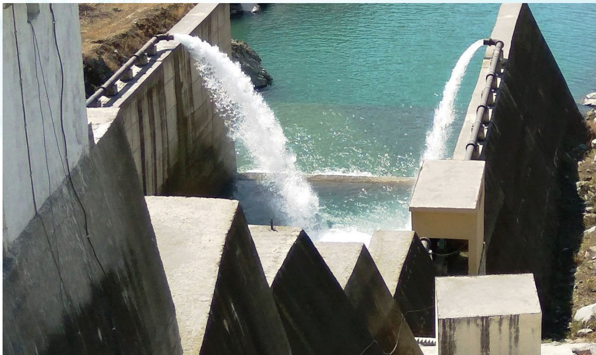
Figure 4.24: E-Flow provision at Parbati-III PS, Himachal Pradesh.
