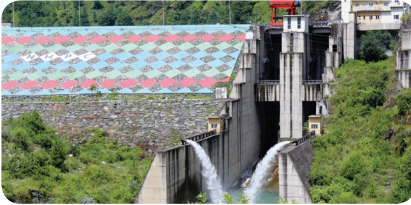
Figure 4.27: Arrangement for e-flow at Parbati-III PS, Himachal Pradesh.
