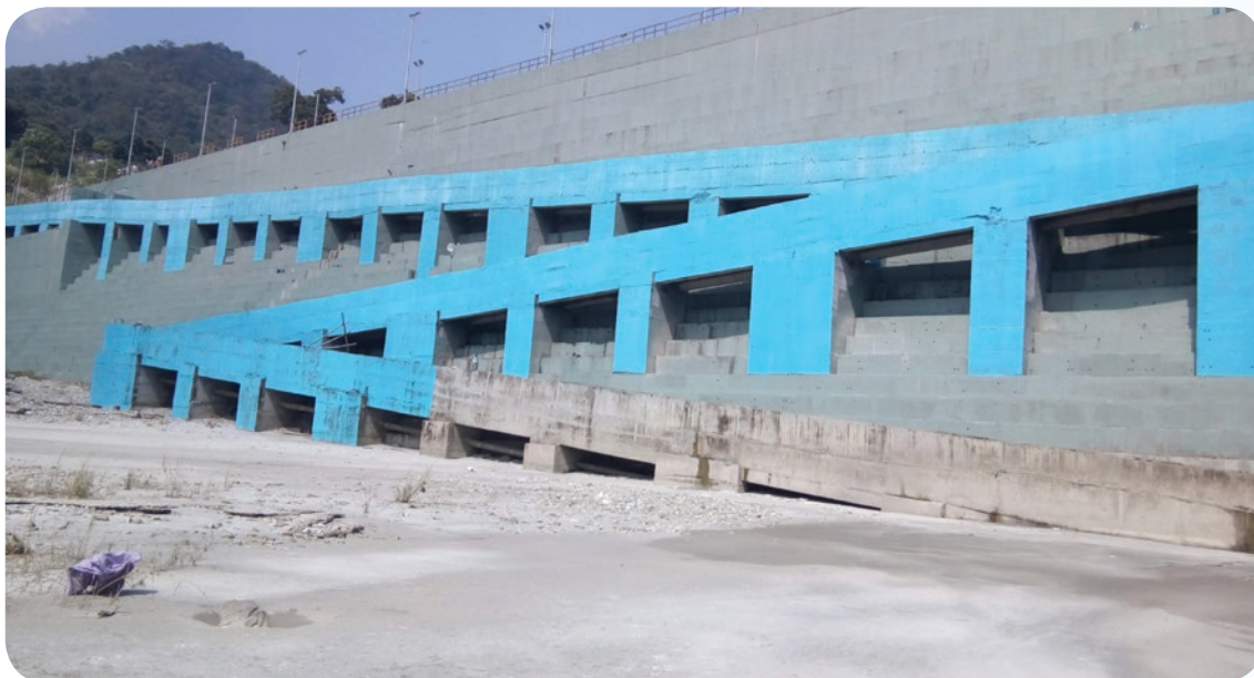
Figure 4.25: Fish ladder along a RCC dam at TLD-IV PS, West Bengal
