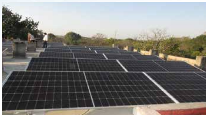
Construction of 150 KVA solar plant
