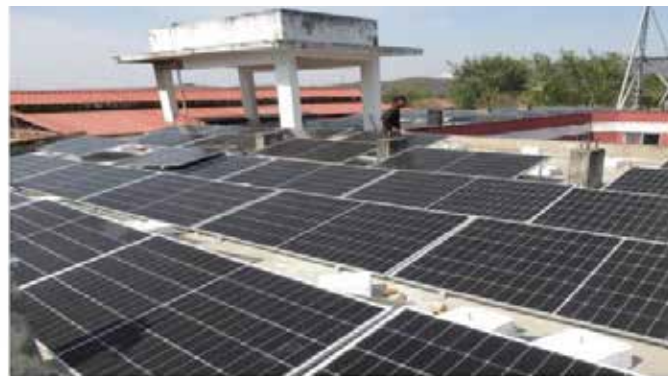
Construction of 150 KVA solar plant
