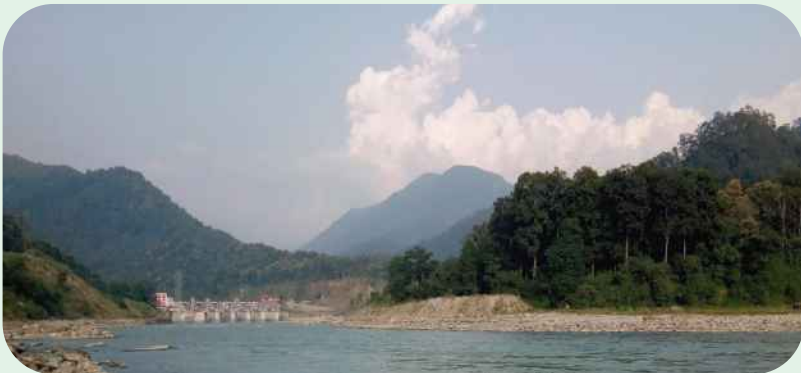
Downstream of TLD-III Power Station (132 MW), West Bengal
