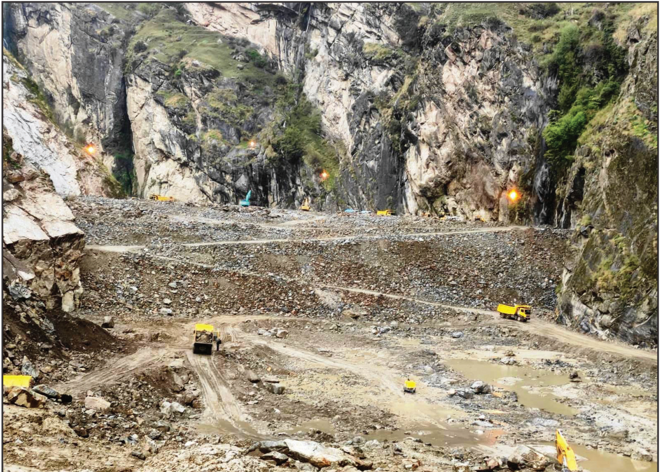
CFRD Dam Filling
