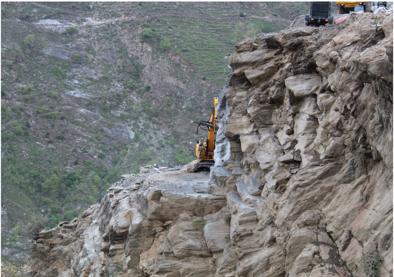
Dam Abutment Stripping
