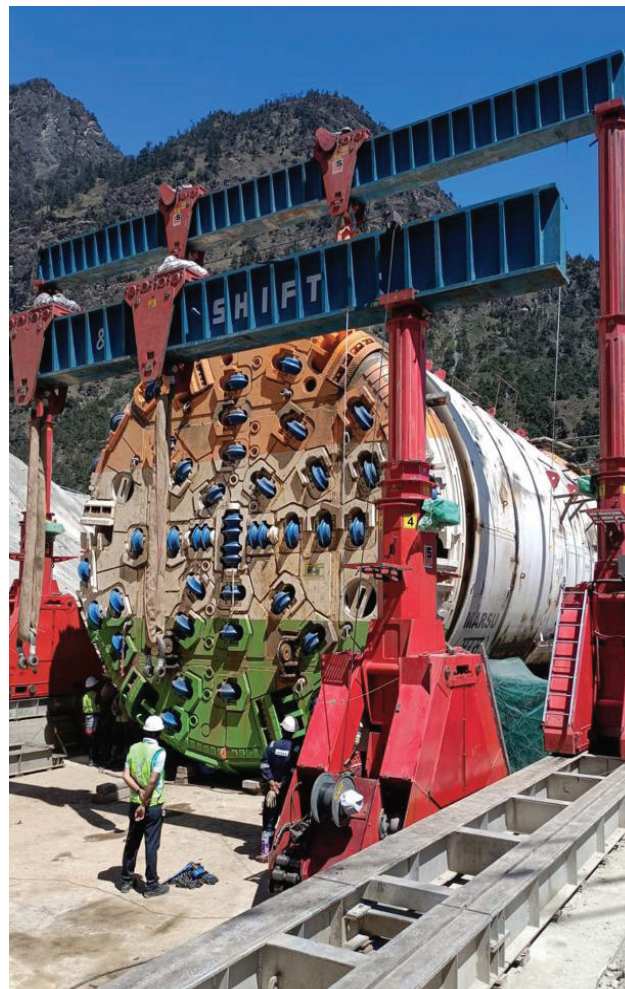
TBM-1 Assembly
