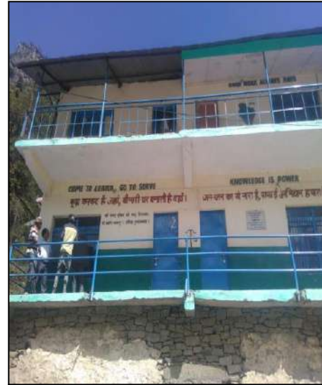
Construction of School Building
