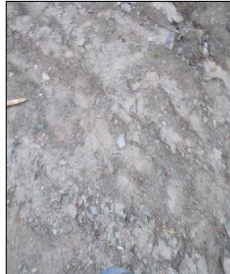
Leveling work @ School Ground
