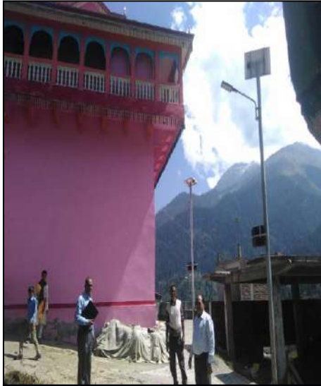
Solar Street Lights under CSR
