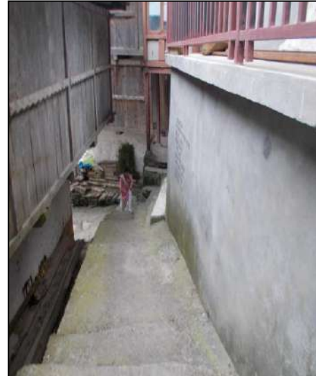
Footpath @ Village Railla
