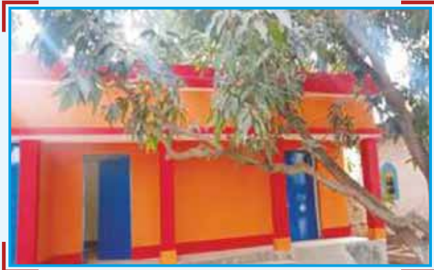
Community centre cum marriage hall constructed at Village:- Benwaliya, Block-Shahpur, Bhojpur, Bihar
