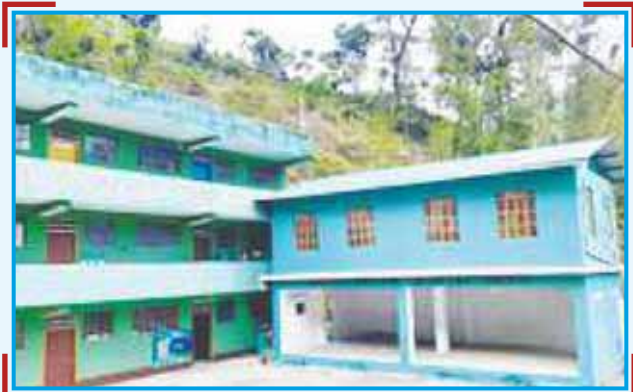
Rangit Power Station Construction of Multipurpose Hall at Legship Village in West Sikkim.
