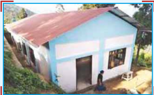
Community Hall along with kitchen & toilet constructed by TLD-III PS at 74 Dhura, Mungpoo, to enable the Villagers to organize community gatherings like meetings, marriages, religious functions, etc
