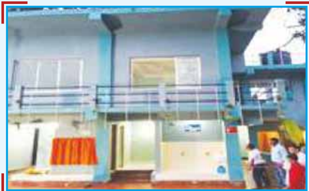
RO-Cum-Sanitation Complex constructed at Gerukamukh and Narayanpu by Subansiri lower HE Project.
