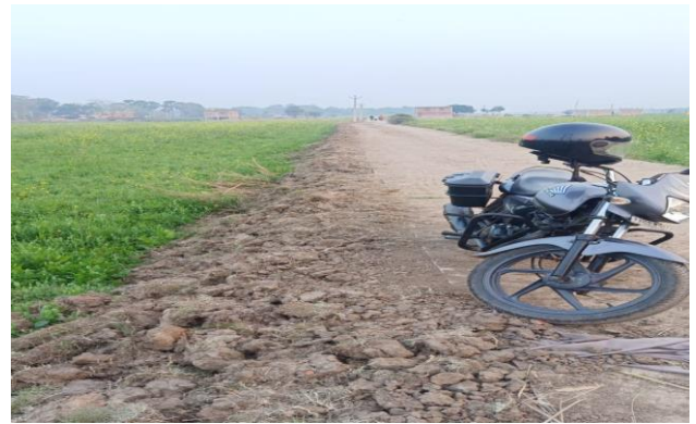
Berm Protection of PCC roads constructed in different villages of Shahpur Block.
