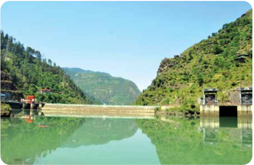
View of Parbati-III Power Station (Dam)
