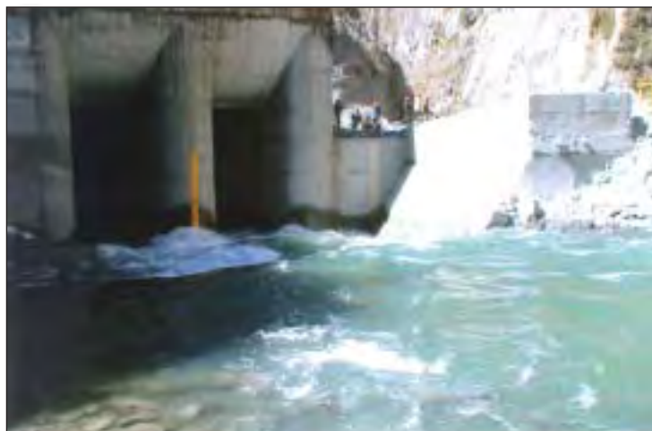
231 MW Chamera - III Project (Himachal Pradesh) - Inlet of Diversion Tunnel
