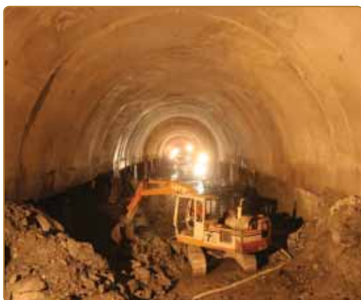
520 MW Parbati-III Project (Himachal Pradesh) - Diversion Tunnel under construction
